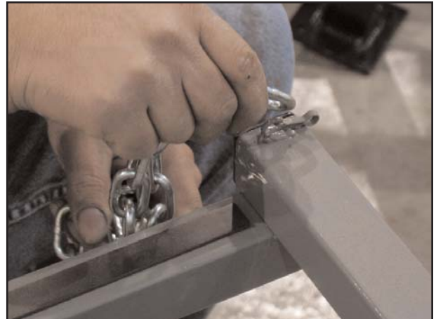
Insert Chain (I) into hook on side of Panel Rest (D). Repeat on other side of Panel Rest (D) with second Chain (I).
