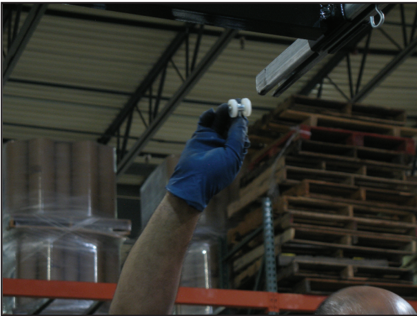
Be sure to insert curtain rollers into curtain rails before installing the last corner rail.
