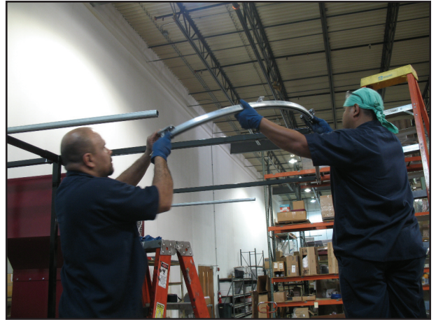
Install the front curtain rail by sliding the rails through the curtain rail supports. Then install the curved curtain rail to the front curtain rail and to the side curtain rail.
